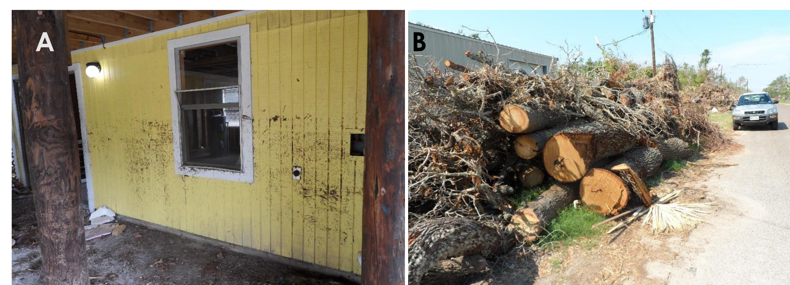
Fig 3. (A) Many houses sustained significant flooding damage. (B) Downed trees soon after their removal from a road. Photos by Kate de Gennaro.
